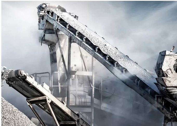
CONVEYOR BELTS AND MATERIAL TRANSFER POINTS
