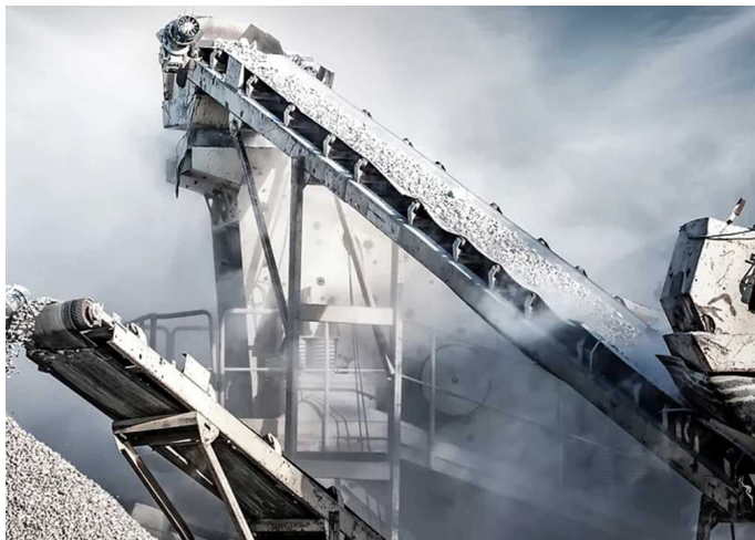
CONVEYOR BELTS AND MATERIAL TRANSFER POINTS
